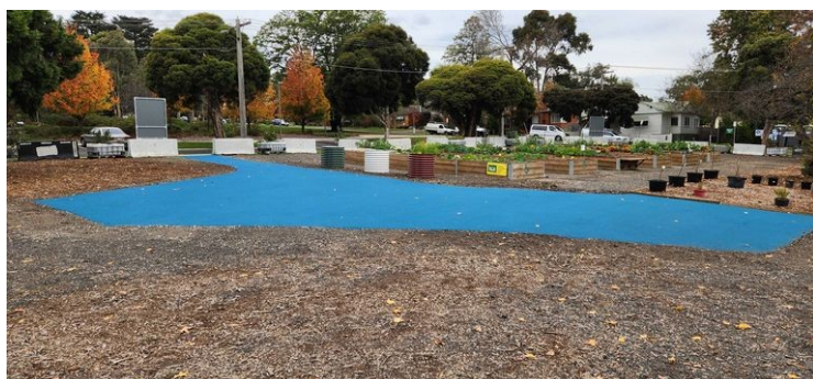
Wheelchair accessible rubber path in preparation for accessible garden beds and bench
